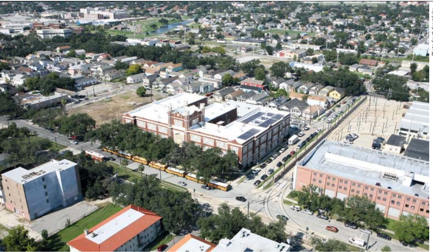
Photo: South Coast Solar
