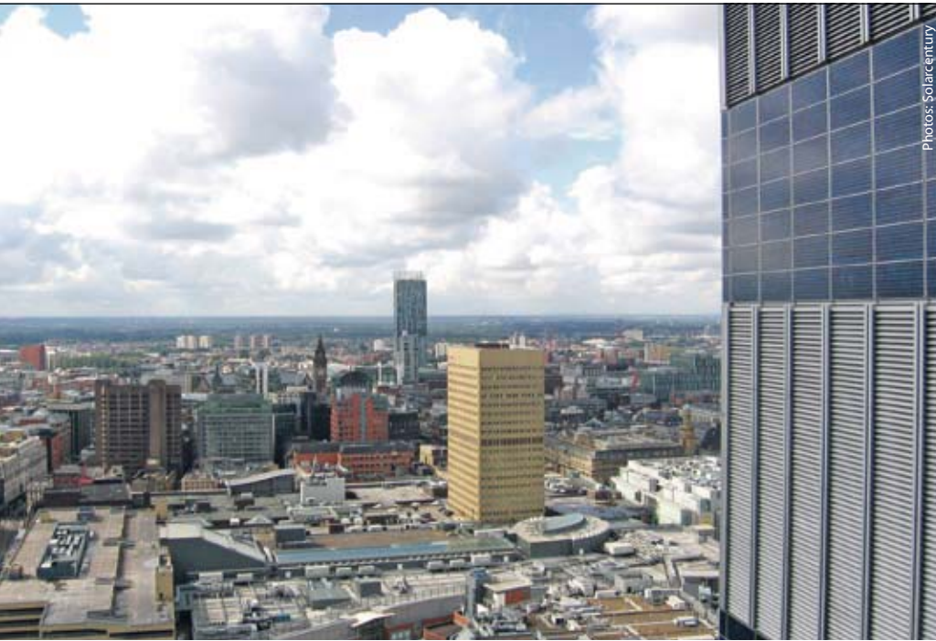
Visionary: The CIS Tower in Manchester, England, a noted local landmark, is clad with photovoltaic panels. The PV modules that cover the tower's entire surface generate 180,000 kilowatt-hours per year.
